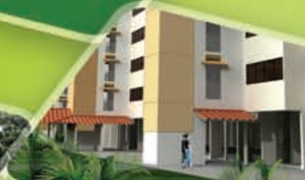
New Lift Shaft
