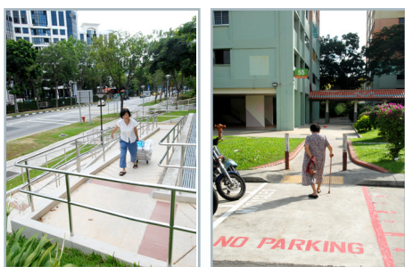
Barrier-free access from block to roadside footpath and car park
