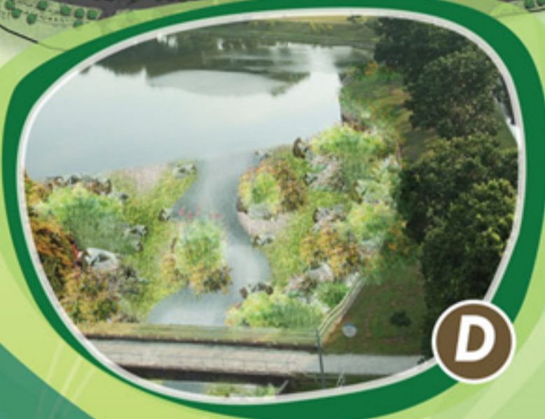
Greening the Spillway with boulders and vegetation for a more natural look.
