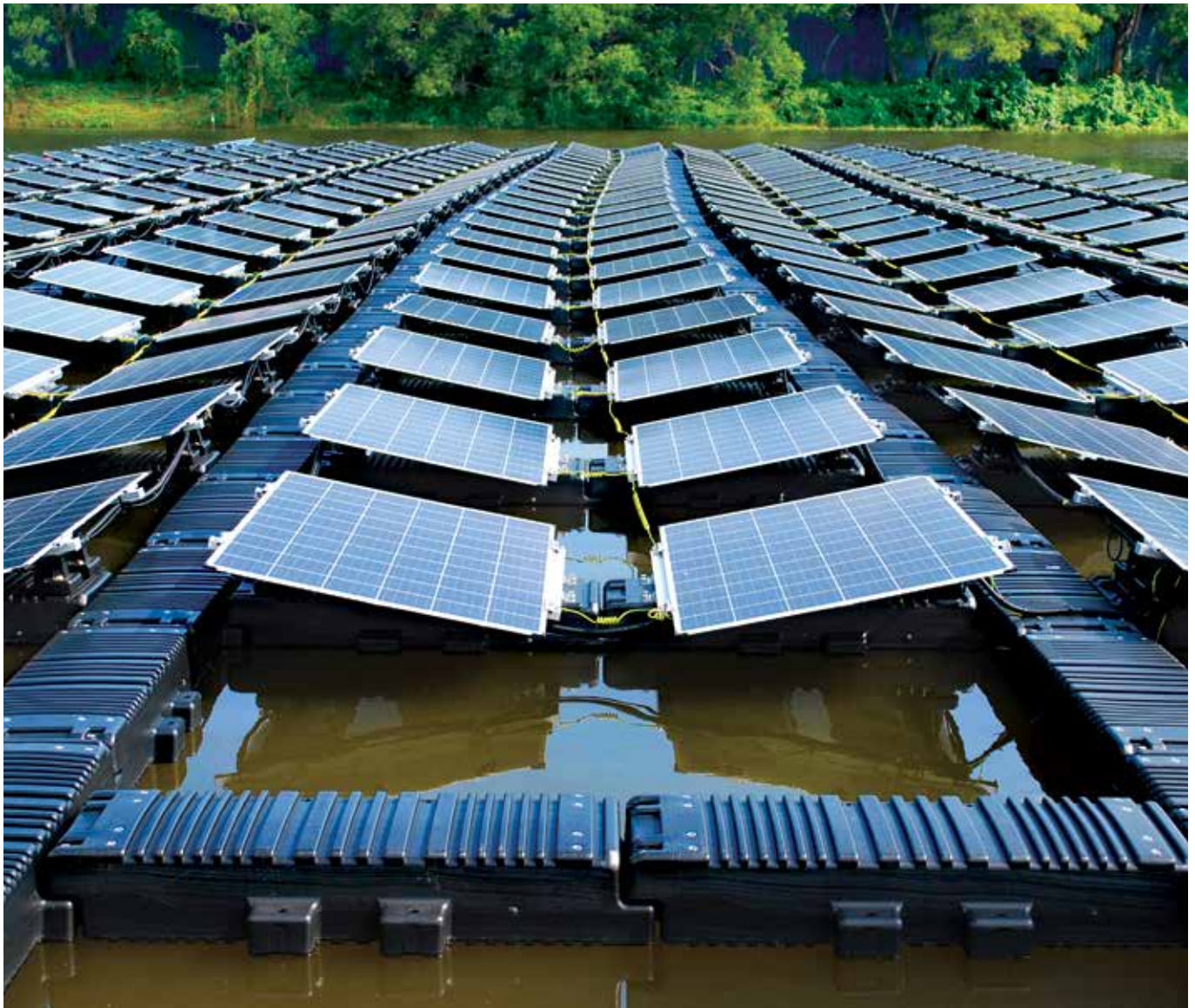
HDB expanded use of its floating system for solar panels in open sea
