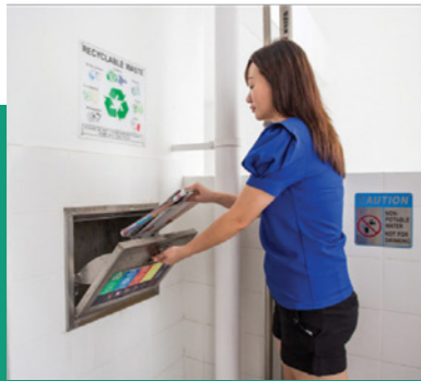
SEPARATE CHUTES FOR RECYCLABLE WASTE
