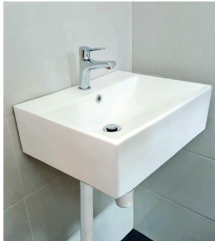
Wash basin with tap mixer
