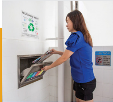
SEPARATE CHUTES FOR RECYCLABLE WASTE
