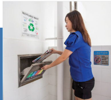
SEPARATE CHUTES FOR RECYCLABLE WASTE
