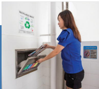
SEPARATE CHUTES FOR RECYCLABLE WASTE
