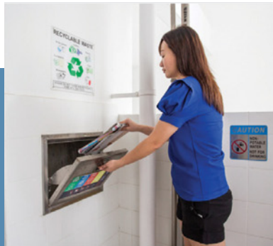
SEPARATE CHUTES FOR RECYCLABLE WASTE
