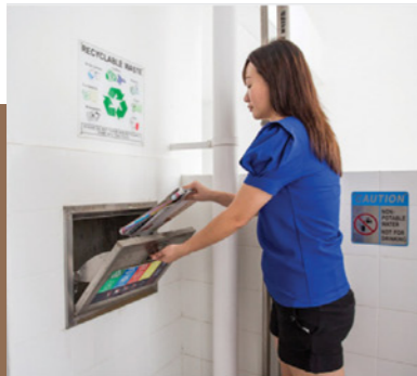
SEPARATE CHUTES FOR RECYCLABLE WASTE
