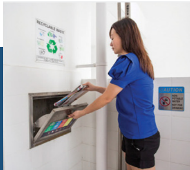
SEPARATE CHUTES FOR RECYCLABLE WASTE
