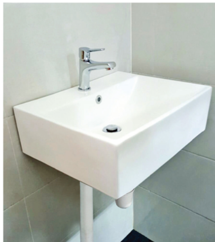
Wash basin with tap mixer
