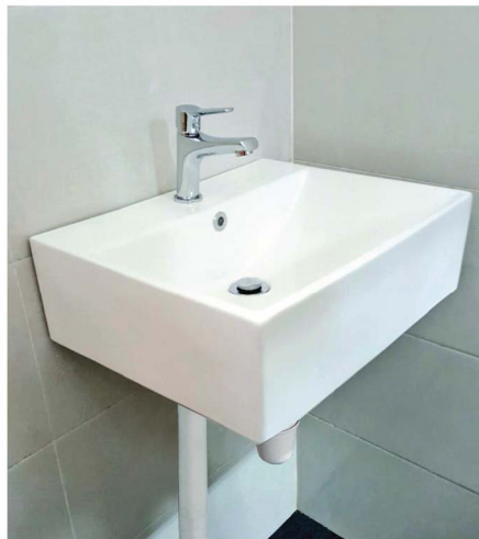
Wash basin with tap mixer
