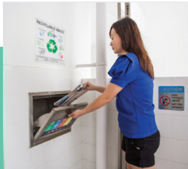
SEPARATE CHUTES FOR RECYCLABLE WASTE
