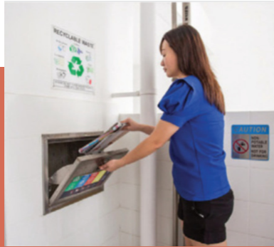
SEPARATE CHUTES FOR RECYCLABLE WASTE
