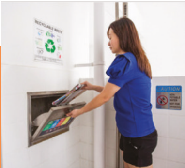
SEPARATE CHUTES FOR RECYCLABLE WASTE
